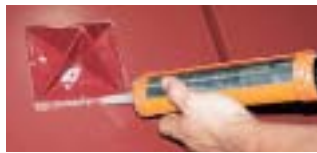
4) Apply bead of sealant around SNO-GEM perimeter.
