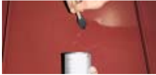
1) After applying thin coat of primer to roof surface.
