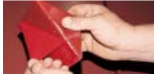
2) Peel release paper backing off adhesive tape on snow guard base.
