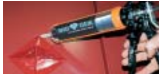
4) Apply bead of sealant around SNO-GEM perimeter.
