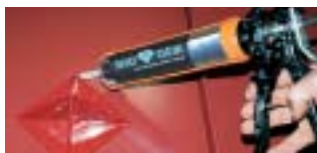
4) Apply bead of sealant around SNO-GEM perimeter.
