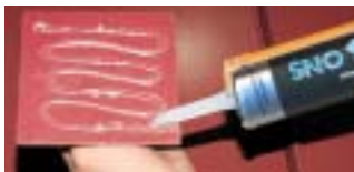
1) Apply sealant bead across SNO-GEM surface.
