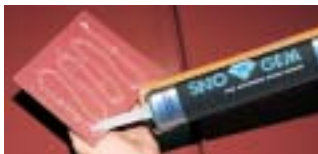
1) Apply sealant bead across SNO-GEM surface and spread evenly.
