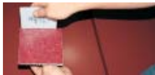
2) Spread sealant evenly before placing snow guard in position on metal surface.
