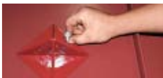
3) Install screws with neoprene gasket washers through pilot holes.
